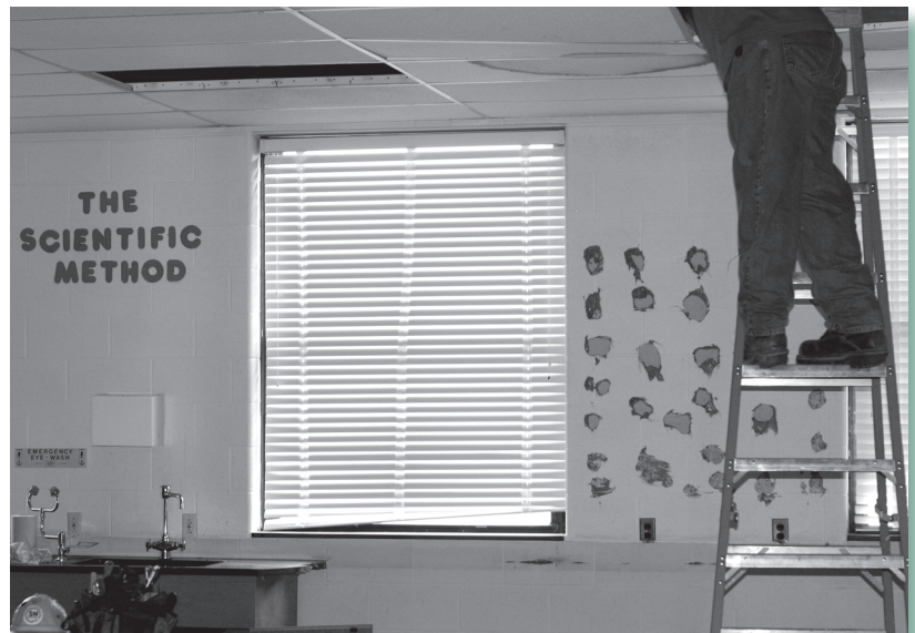
This past summer, several classrooms were renovated at Roth Middle School. Improvements will continue to be made to the school throughout much of 2008.
