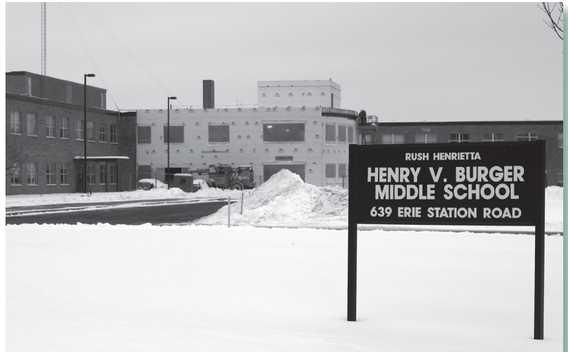
A new addition near the existing bus loop is one of the many enhancements taking place at Burger Middle School. Rush-Henrietta voters approved the work in December 2005.
